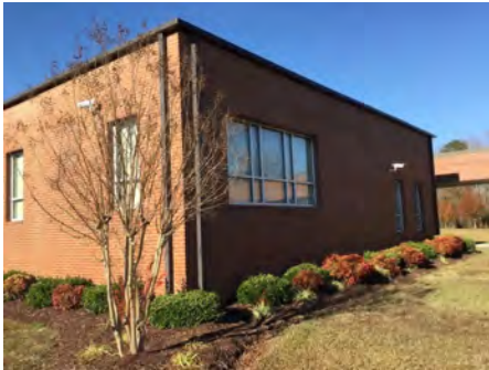
4). East Elevation - Dec 08, 2016
