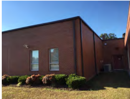
5). North Elevation - Dec 08, 2016
