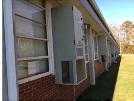
2). East Elevation - Dec 08, 2016
