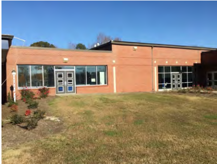
1). South Elevation - Dec 08, 2016
