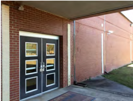
4). East Elevation - Dec 08, 2016
