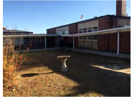
3). North Elevation - Dec 08, 2016
