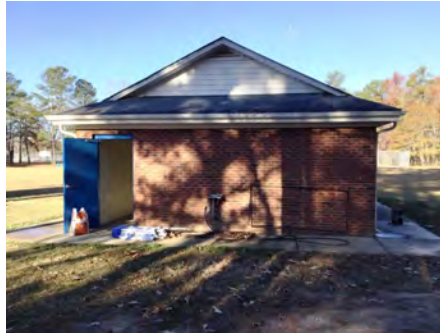
2). East Elevation - Dec 06, 2016
