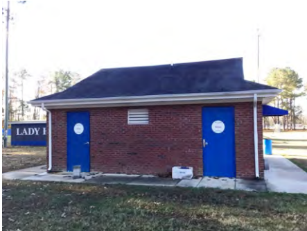
1). North Elevation - Dec 06, 2016
