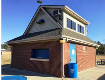
2). Northeast Elevation - Dec 06, 2016
