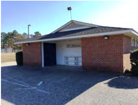
4). North Elevation - Dec 06, 2016
