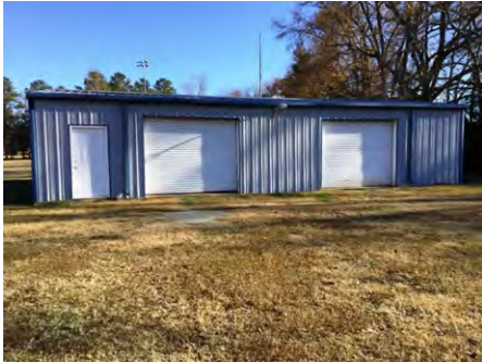
1). Southwest Elevation - Dec 07, 2016
