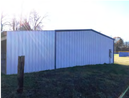
4). Northwest Elevation - Dec 07, 2016
