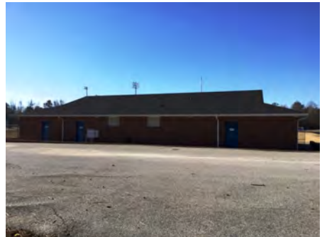
3). East Elevation - Dec 06, 2016
