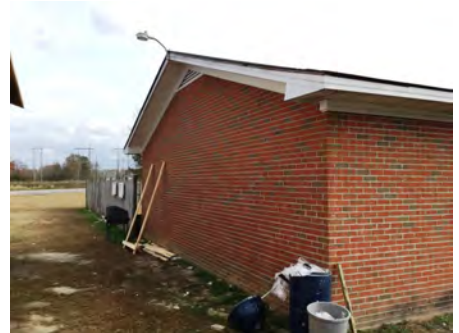
3). Northwest Elevation - Dec 07, 2016
