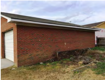
4). East Elevation - Dec 07, 2016
