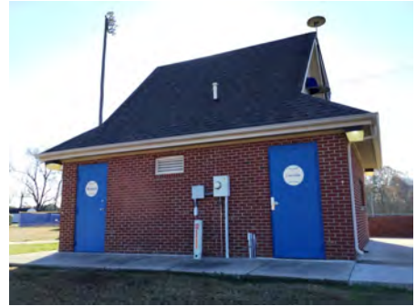
3). North Elevation - Dec 06, 2016
