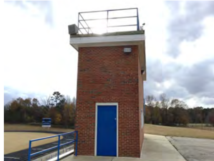
2). East Elevation - Dec 06, 2016
