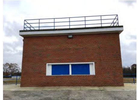
3). North Elevation - Dec 06, 2016
