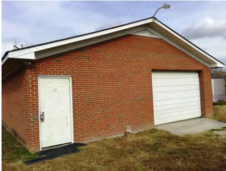
1). South Elevation - Dec 07, 2016
