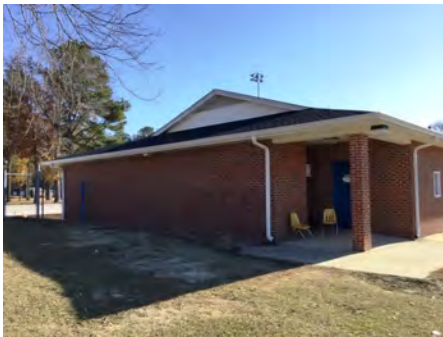
4). North Elevation - Dec 06, 2016
