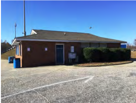
1). East Elevation - Dec 06, 2016
