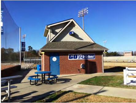
1). East Elevation - Dec 06, 2016
