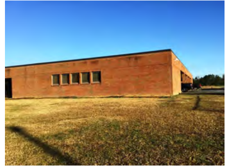
3). East Elevation - Dec 05, 2016
