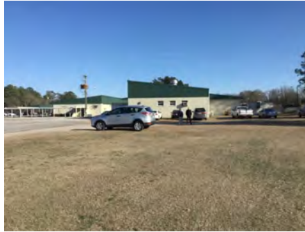
2). Northwest Elevation - Feb 21, 2017
