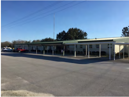
1). Northeast Elevation - Feb 21, 2017
