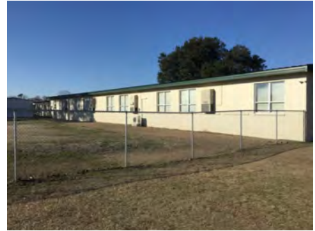
3). Southwest Elevation - Feb 21, 2017
