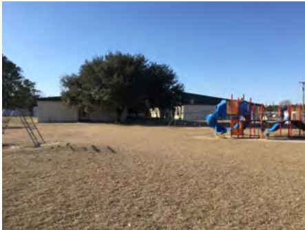
4). Southeast Elevation - Feb 21, 2017
