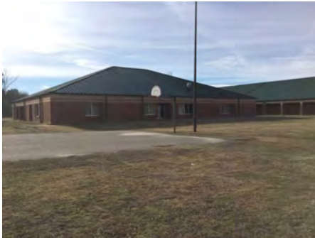
4). North Elevation - Jan 11, 2017
