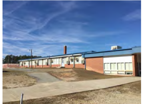
3). South Elevation - Mar 03, 2017
