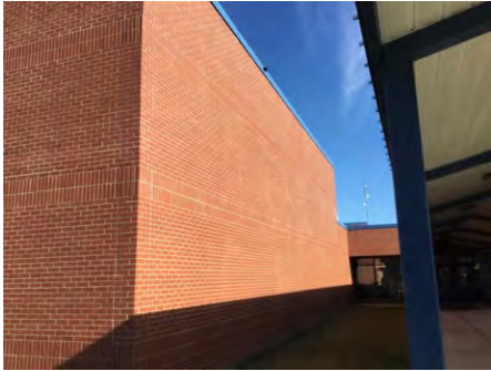
1). South Elevation - Mar 03, 2017
