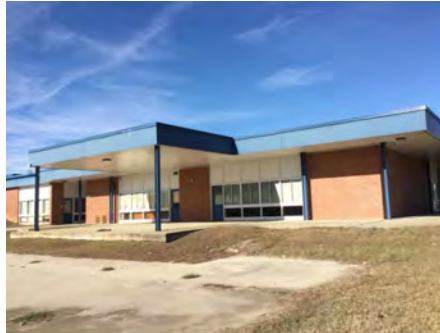
2). South Elevation - Mar 03, 2017
