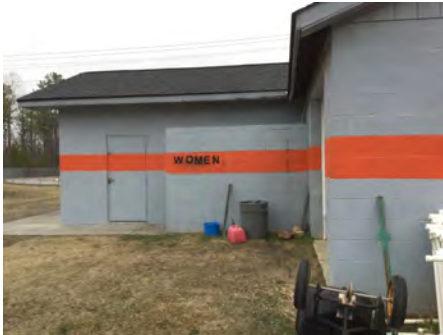
4). Southwest Elevation - Jan 23, 2017
