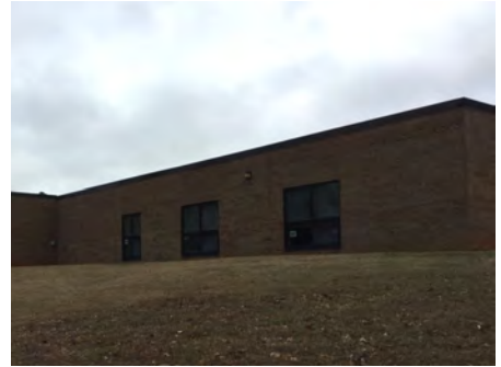
3). Northwest Elevation - Jan 23, 2017
