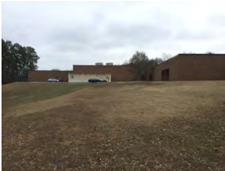
4). Northwest Elevation - Jan 25, 2017
