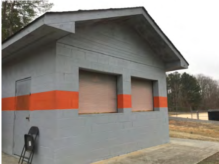
1). Northwest Elevation - Jan 23, 2017
