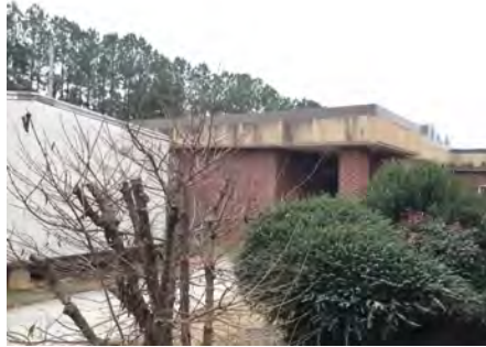
2). North Elevation - Jan 23, 2017
