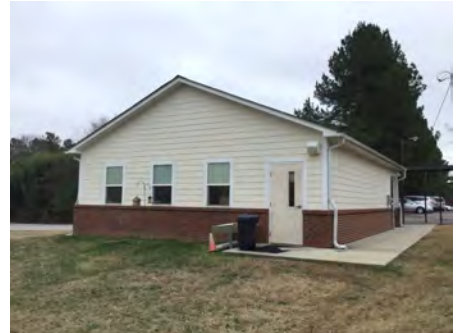
3). North Elevation - Jan 23, 2017
