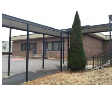
2). Northeast Elevation - Jan 23, 2017
