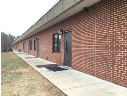
1). Northwest Elevation - Jan 23, 2017
