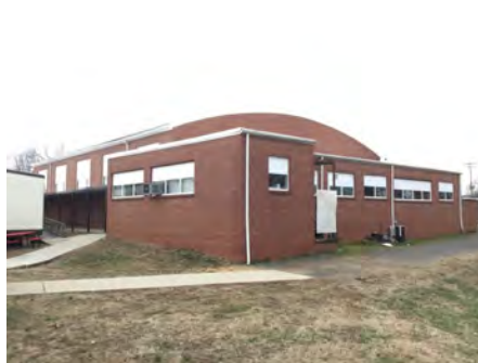
5). North Elevation - Jan 23, 2017
