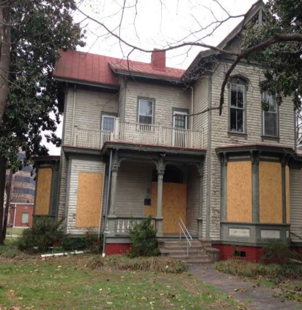
Unused boarded-up home allocated to the Department of Administration
