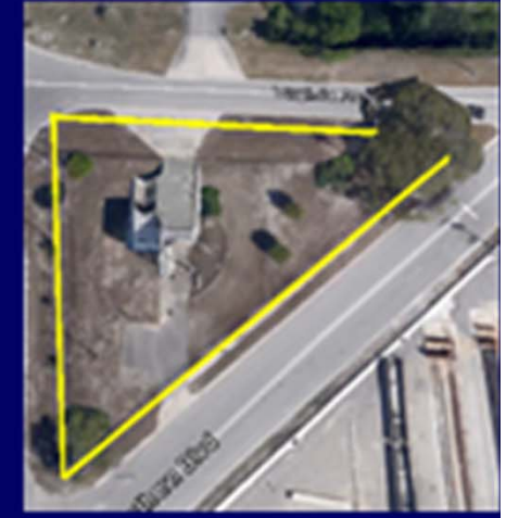
Gas and Calibration Station
