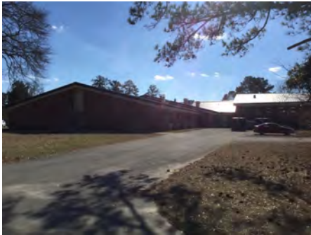
4). Northeast Elevation - Feb 15, 2017
