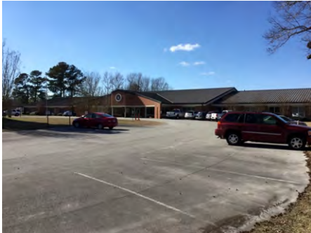
1). Southeast Elevation - Feb 15, 2017
