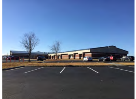
3). Northeast Elevation - Dec 05, 2016
