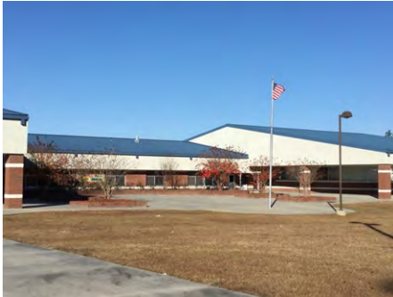
1). East Elevation - Dec 05, 2016
