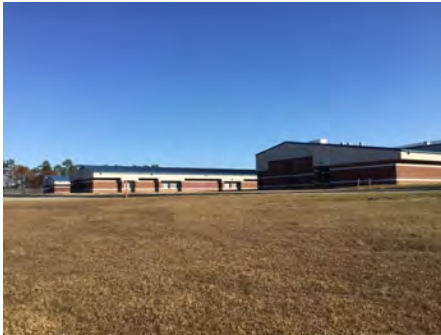
4). Southwest Elevation - Dec 05, 2016
