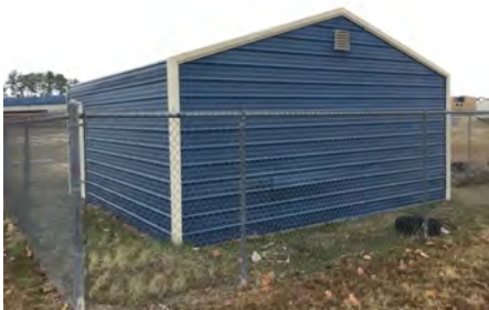
4). Northwest Elevation - Dec 05, 2016
