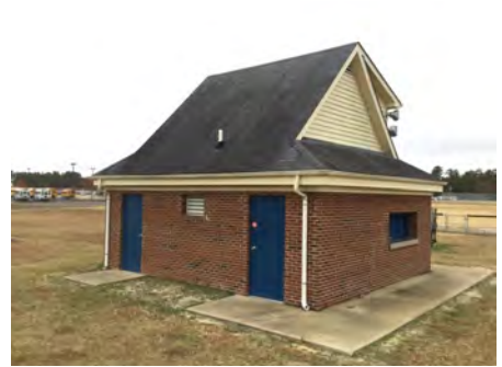
3). Northeast Elevation - Dec 05, 2016
