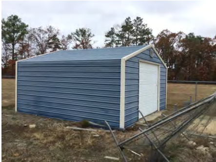
1). Southwest Elevation - Dec 05, 2016
