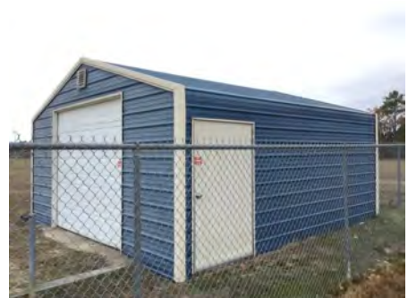
3). Northeast Elevation - Dec 05, 2016
