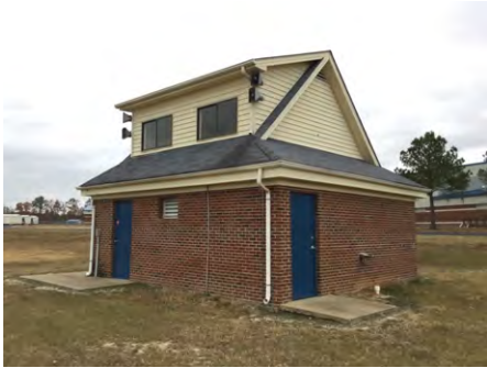
1). Southwest Elevation - Dec 05, 2016
