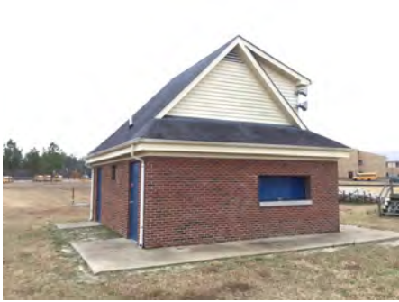
4). Northwest Elevation - Dec 05, 2016
