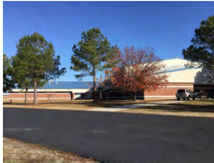
5). South Elevation - Dec 05, 2016
