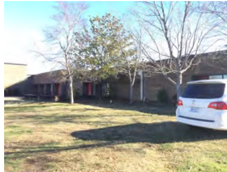
5). Southwest Elevation - Feb 10, 2017
