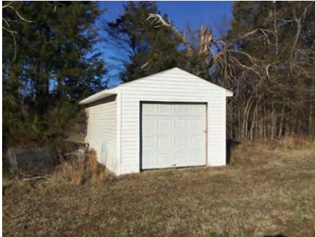
1). East Elevation - Feb 10, 2017
