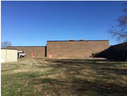
4). Southwest Elevation - Feb 10, 2017
