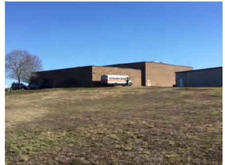
3). West Elevation - Feb 10, 2017
