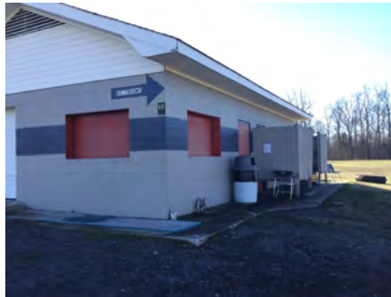
2). Northwest Elevation - Feb 10, 2017
