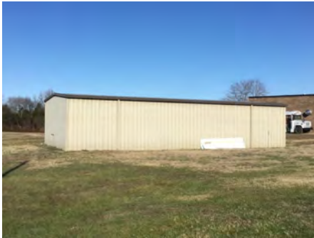
4). Southeast Elevation - Feb 10, 2017
