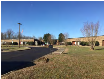
1). East Elevation - Feb 10, 2017
