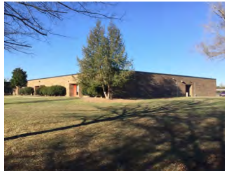
2). North Elevation - Feb 10, 2017
