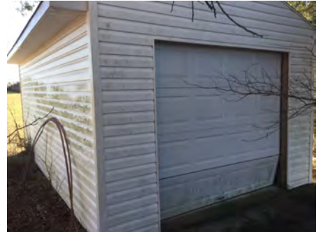
3). Northwest Elevation - Feb 10, 2017
