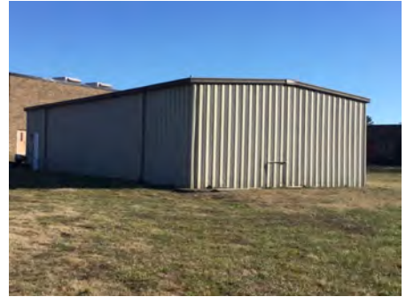
3). Southwest Elevation - Feb 10, 2017
