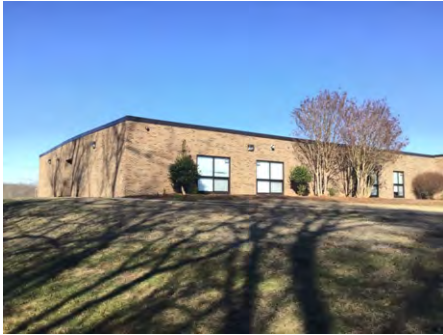
1). East Elevation - Feb 10, 2017
