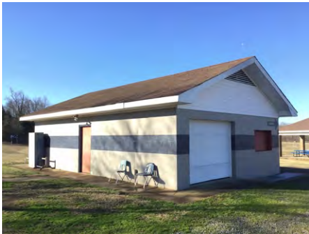
1). Northeast Elevation - Feb 10, 2017
