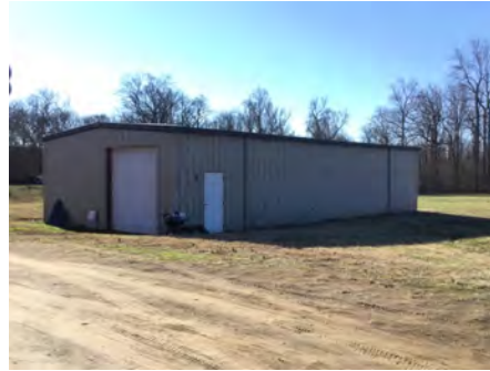
2). Northwest Elevation - Feb 10, 2017
