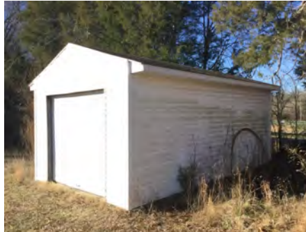
2). Northeast Elevation - Feb 10, 2017
