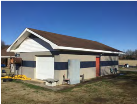
4). Southeast Elevation - Feb 10, 2017
