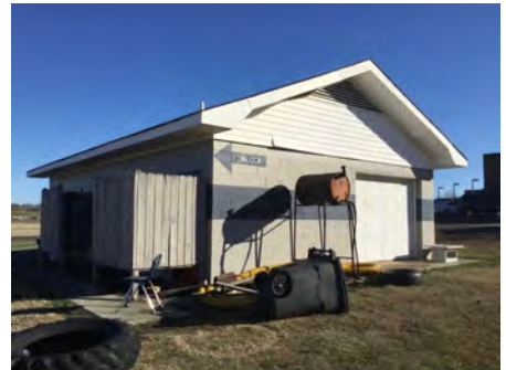
3). Southwest Elevation - Feb 10, 2017
