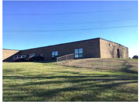
3). West Elevation - Feb 10, 2017
