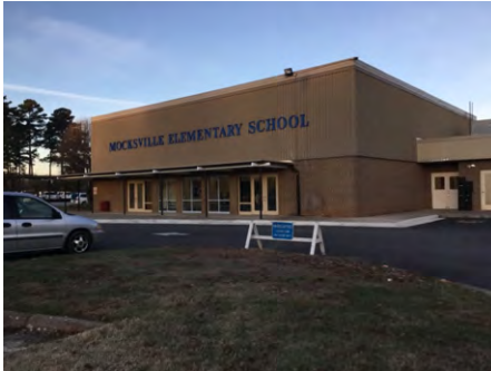
1). East Elevation - Mar 06, 2017
