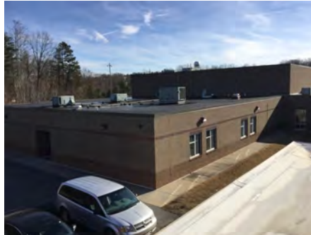
2). Southwest Elevation - Feb 13, 2017
