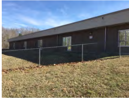
2). Northwest Elevation - Feb 13, 2017
