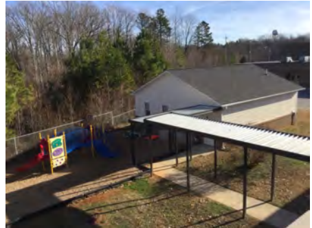
3). Northwest Elevation - Feb 13, 2017
