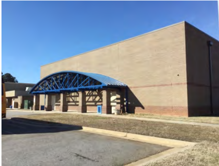
1). Southeast Elevation - Feb 13, 2017
