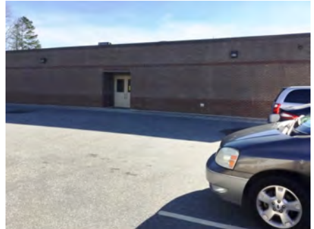
3). Northwest Elevation - Feb 13, 2017
