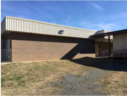
1). Southwest Elevation - Feb 13, 2017
