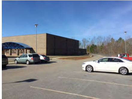
2). North Elevation - Mar 06, 2017
