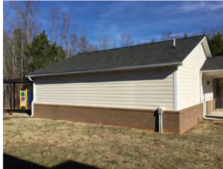
2). Southwest Elevation - Feb 13, 2017
