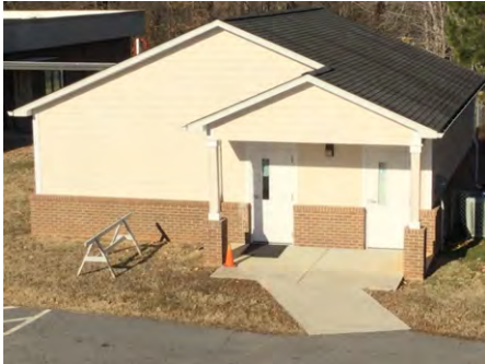
1). Southeast Elevation - Feb 13, 2017
