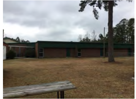
3). North Elevation - Feb 08, 2017
