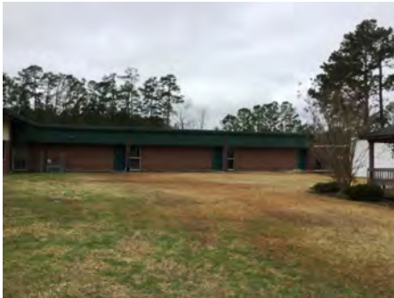
4). East Elevation - Feb 08, 2017
