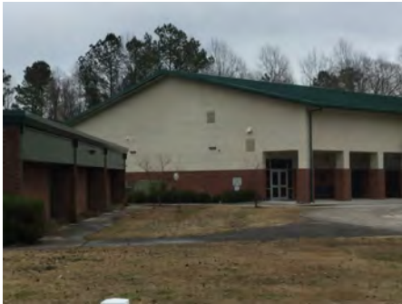
4). Northwest Elevation - Feb 08, 2017
