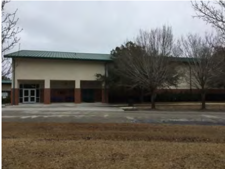
1). Southwest Elevation - Feb 08, 2017
