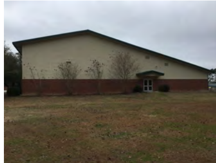
2). Southeast Elevation - Feb 08, 2017
