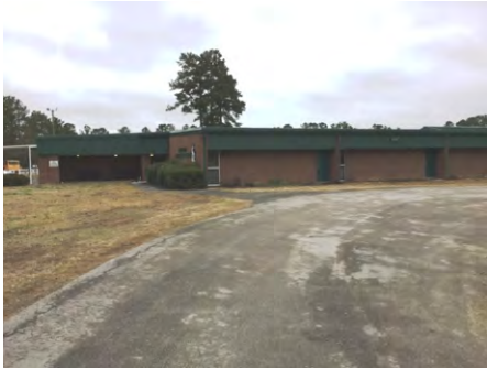
1). South Elevation - Feb 08, 2017
