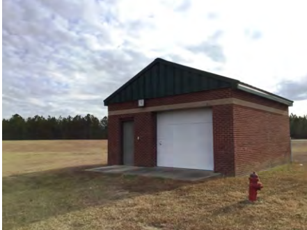
1). Northeast Elevation - Nov 28, 2016
