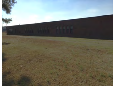
2). East Elevation - Dec 07, 2016
