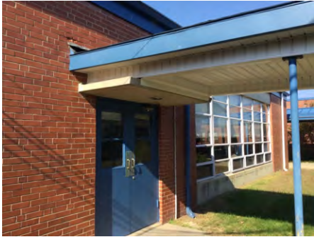
1). North Elevation - Dec 06, 2016
