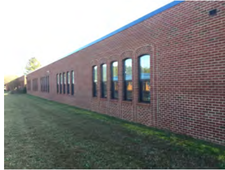
2). North Elevation - Dec 07, 2016
