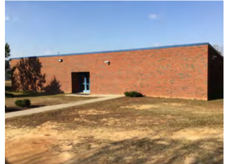
3). South Elevation - Dec 07, 2016
