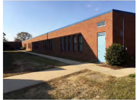
3). South Elevation - Dec 07, 2016
