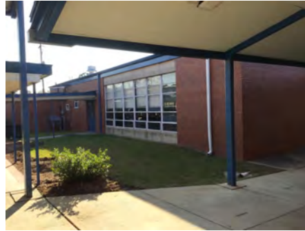
2). East Elevation - Dec 06, 2016
