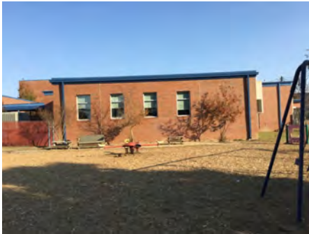
4). South Elevation - Dec 06, 2016
