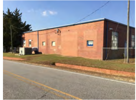
3). South Elevation - Dec 07, 2016
