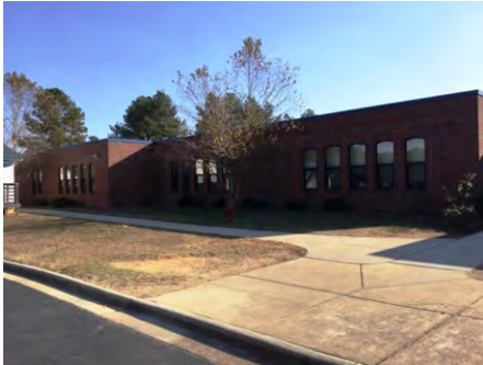
1). North Elevation - Dec 07, 2016
