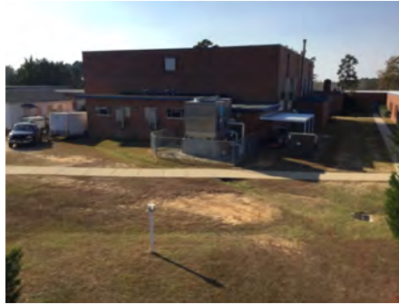
2). East Elevation - Dec 07, 2016
