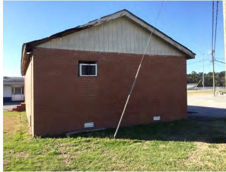
2). North Elevation - Feb 20, 2017
