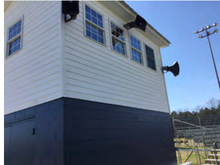
2). Northwest Elevation - Feb 21, 2017
