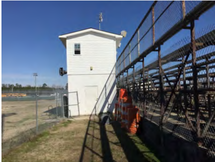
1). South Elevation - Feb 21, 2017
