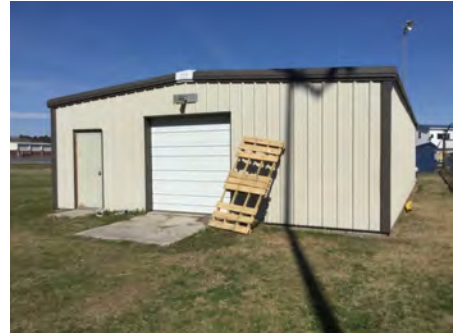
3). Southwest Elevation - Feb 21, 2017
