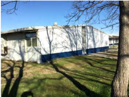
4). East Elevation - Feb 20, 2017
