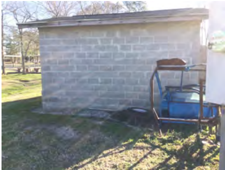
4). West Elevation - Feb 20, 2017
