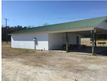
2). East Elevation - Feb 21, 2017
