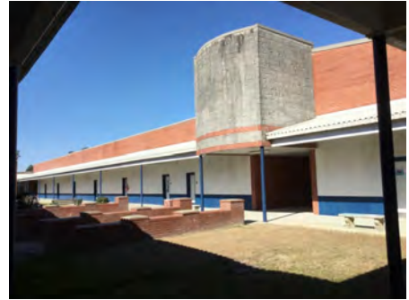
3). South Elevation - Feb 20, 2017
