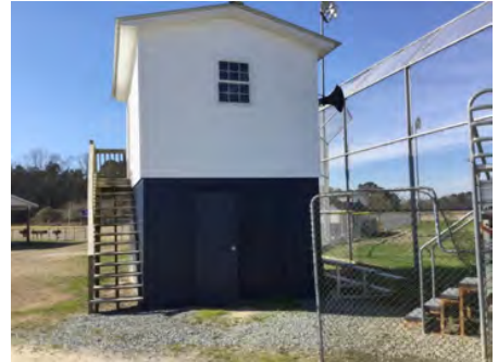
3). Northeast Elevation - Feb 21, 2017
