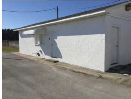
2). East Elevation - Feb 20, 2017
