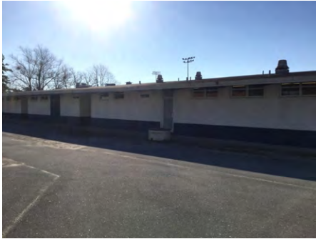
1). North Elevation - Feb 20, 2017
