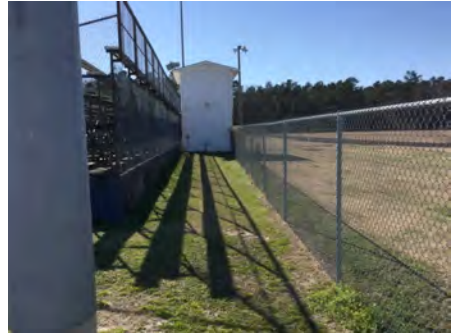
3). North Elevation - Feb 21, 2017
