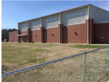
2). East Elevation - Feb 21, 2017
