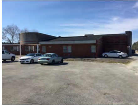
2). East Elevation - Feb 24, 2017
