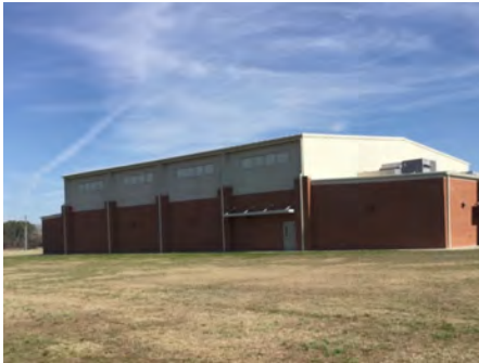
4). West Elevation - Feb 21, 2017
