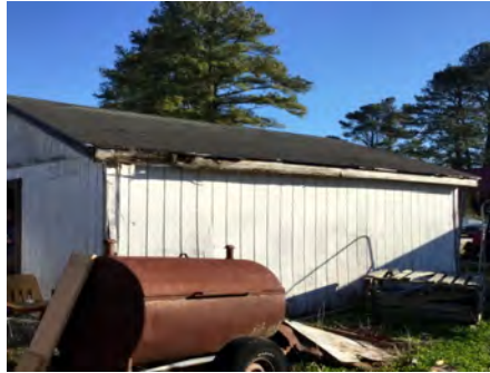
2). South Elevation - Feb 20, 2017
