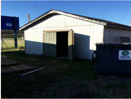
1). West Elevation - Feb 20, 2017
