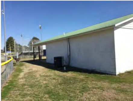
4). West Elevation - Feb 21, 2017
