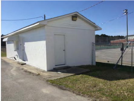
1). North Elevation - Feb 20, 2017
