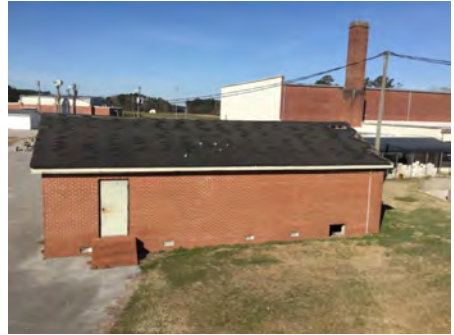
3). West Elevation - Feb 20, 2017
