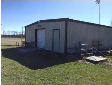
1). Northeast Elevation - Feb 21, 2017
