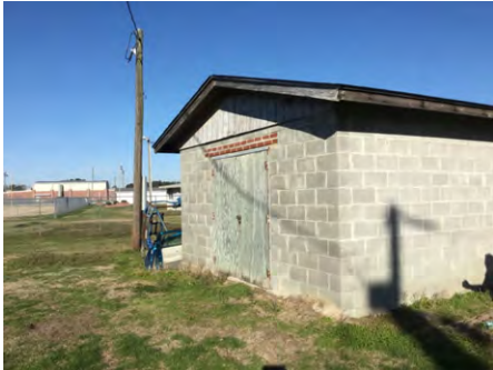
1). South Elevation - Feb 20, 2017
