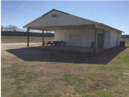
1). North Elevation - Feb 21, 2017
