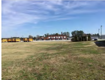
2). West Elevation - Feb 20, 2017
