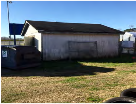
4). North Elevation - Feb 20, 2017
