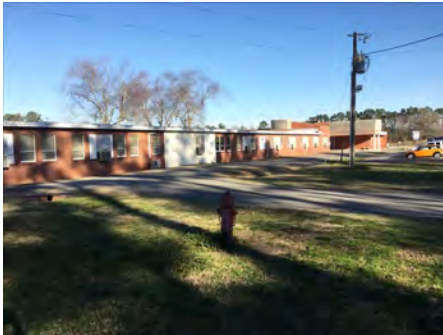
4). East Elevation - Feb 20, 2017
