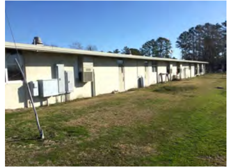
3). South Elevation - Feb 20, 2017
