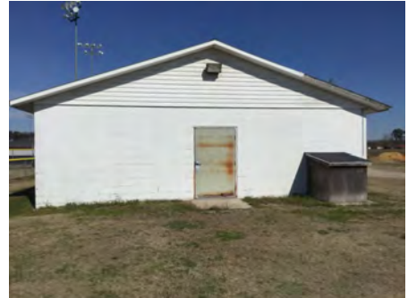
3). South Elevation - Feb 21, 2017
