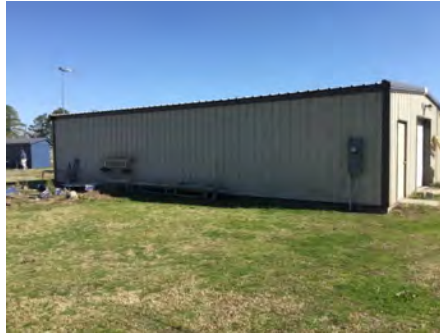
2). Northwest Elevation - Feb 21, 2017
