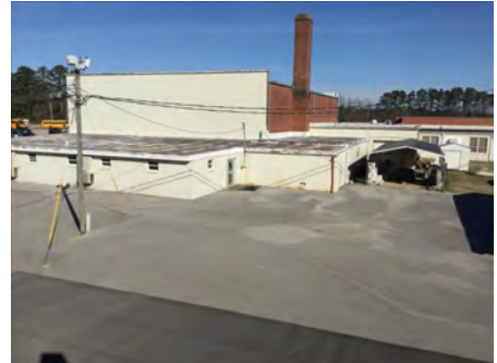
3). Partial South Elevation - Feb 20, 2017
