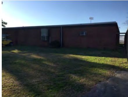
2). North Elevation - Feb 20, 2017
