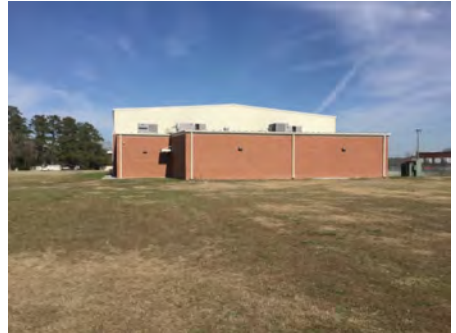
3). South Elevation - Feb 21, 2017
