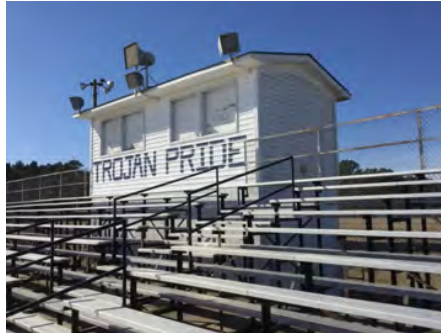
2). East Elevation - Feb 21, 2017
