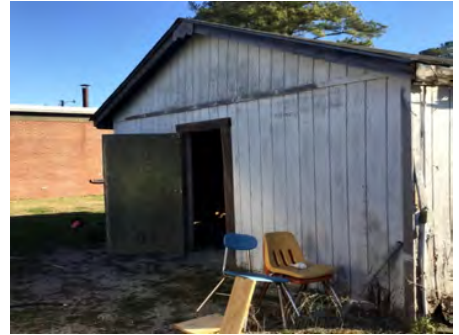
3). East Elevation - Feb 20, 2017
