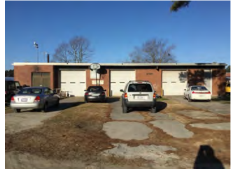
3). East Elevation - Feb 20, 2017
