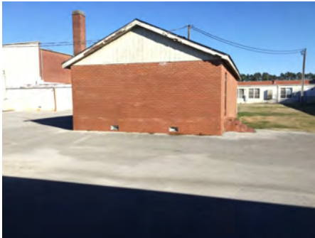
4). South Elevation - Feb 20, 2017
