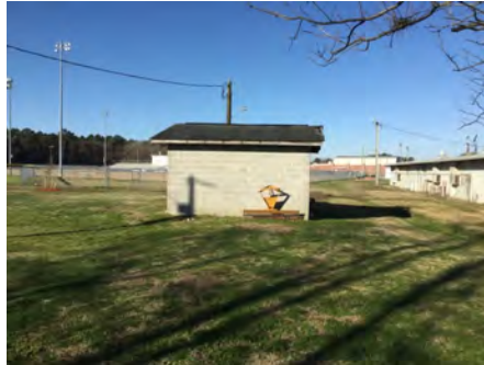
2). East Elevation - Feb 20, 2017
