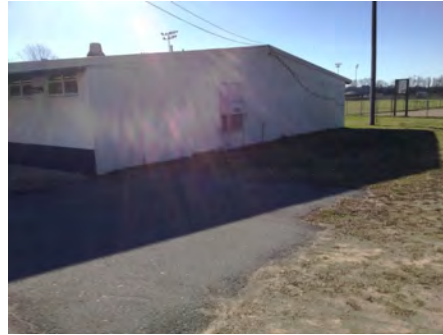
2). West Elevation - Feb 20, 2017
