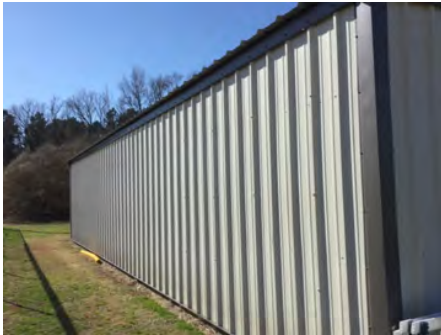
4). Southeast Elevation - Feb 21, 2017
