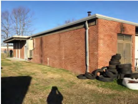
4). South Elevation - Feb 20, 2017
