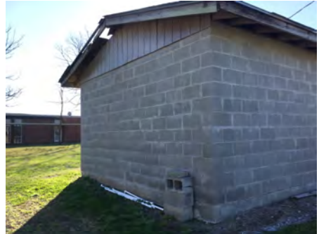
3). North Elevation - Feb 20, 2017
