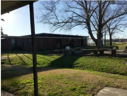
1). West Elevation - Feb 20, 2017
