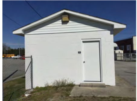
3). South Elevation - Feb 20, 2017
