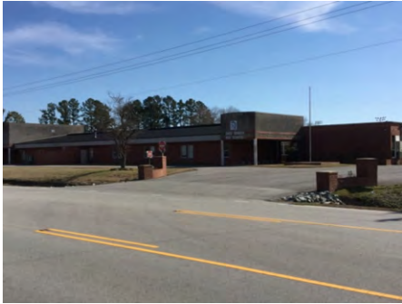
1). Partial North Elevation - Feb 24, 2017
