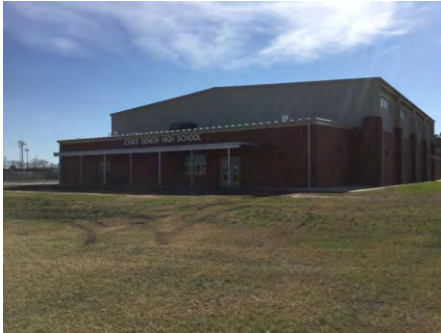
1). North Elevation - Feb 21, 2017
