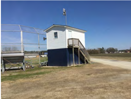
1). Southeast Elevation - Feb 21, 2017
