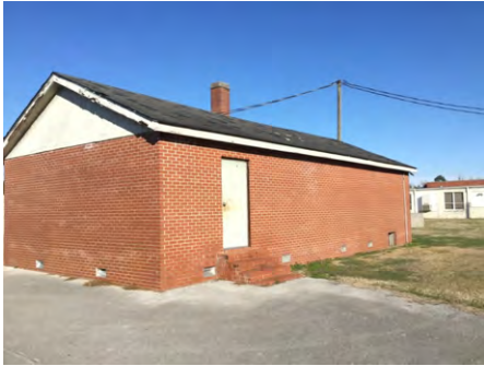
1). East Elevation - Feb 20, 2017
