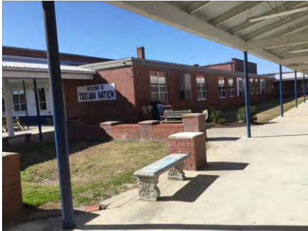
1). North Elevation - Feb 20, 2017
