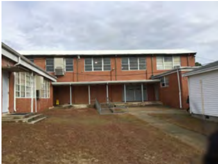
4). South Elevation - Dec 08, 2016
