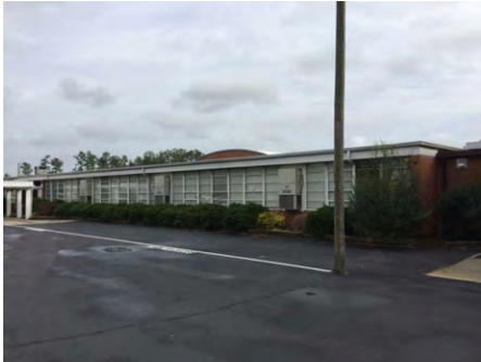
1). West Elevation - Dec 08, 2016
