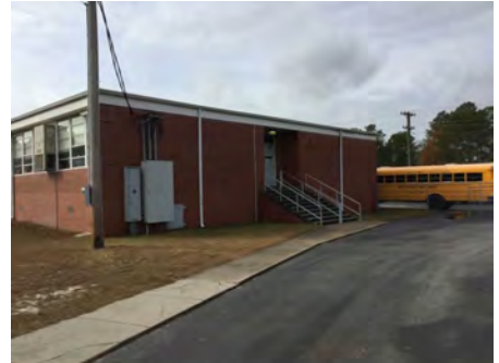
3). North Elevation - Dec 08, 2016
