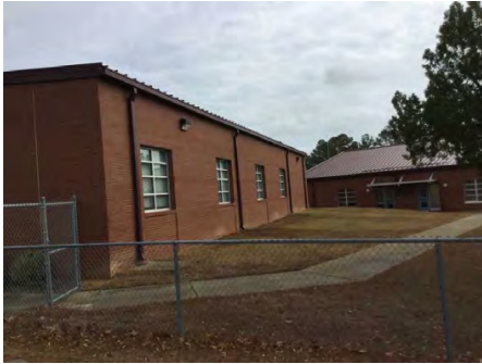
1). South Elevation - Dec 08, 2016
