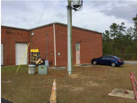
1). East Elevation - Dec 08, 2016
