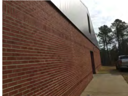
2). South Elevation - Dec 08, 2016
