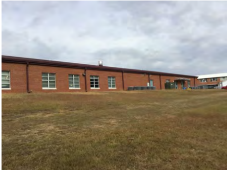
1). East Elevation - Dec 08, 2016
