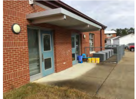
3). North Elevation - Dec 08, 2016
