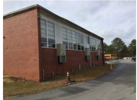
3). North Elevation - Dec 08, 2016
