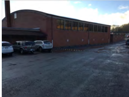
2). Northwest Elevation - Feb 09, 2017
