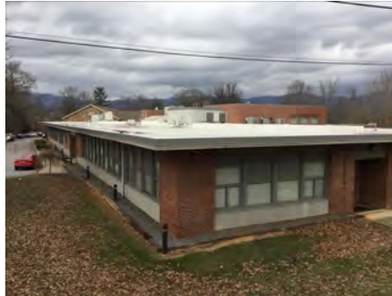
2). Southwest Elevation - Feb 09, 2017
