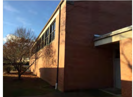
3). East Elevation - Feb 09, 2017
