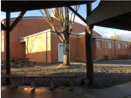
1). North Elevation - Feb 09, 2017
