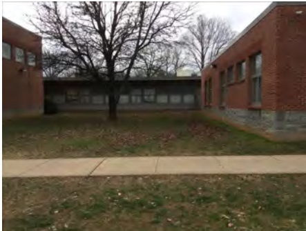
4). East Elevation - Feb 09, 2017
