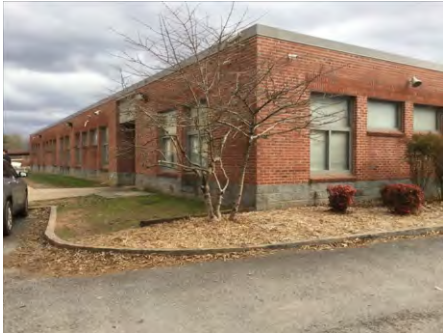
1). North Elevation - Feb 09, 2017
