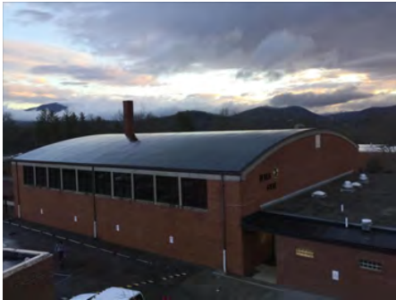
4). Southwest Elevation - Feb 09, 2017
