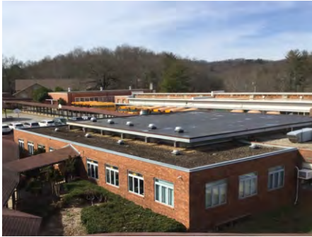
1). South Elevation - Feb 27, 2017
