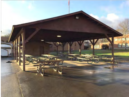
1). North Elevation - Jan 30, 2017
