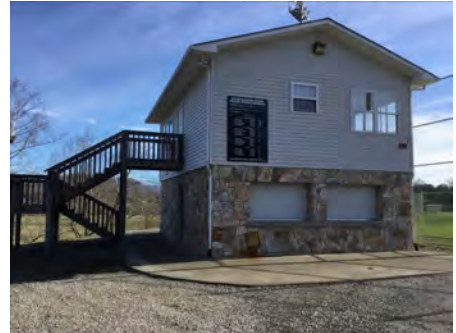
3). Northeast Elevation - Jan 24, 2017
