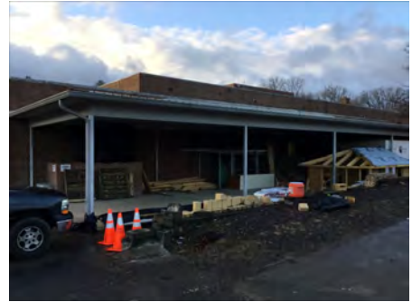
3). North Elevation - Jan 27, 2017
