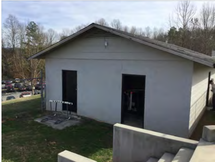
1). North Elevation - Feb 08, 2017
