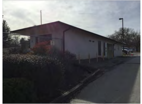
3). North elevation - Jan 30, 2017
