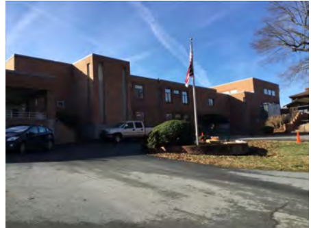
3). North Elevation - Jan 24, 2017
