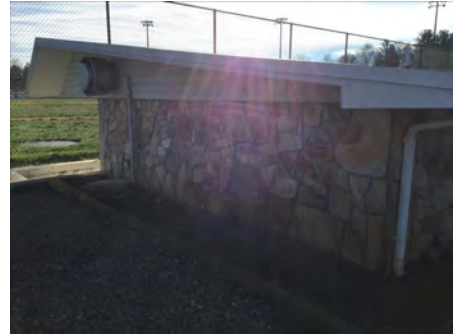
3). North Elevation - Jan 24, 2017
