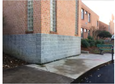
3). North Elevation - Feb 08, 2017
