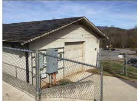
3). South Elevation - Feb 08, 2017
