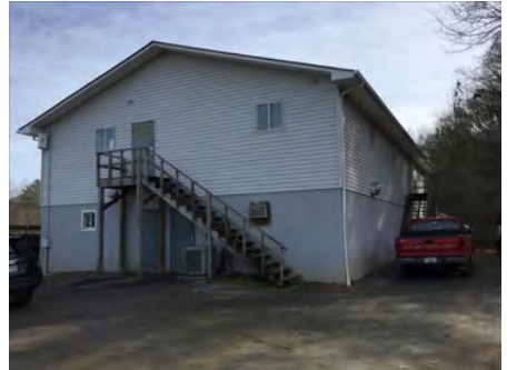
3). Northwest Elevation - Feb 07, 2017
