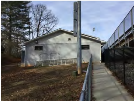
4). South Elevation - Feb 07, 2017
