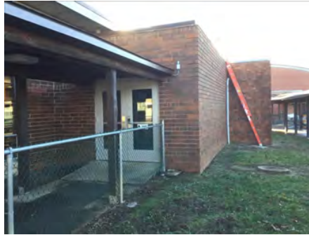
2). West Elevation - Feb 23, 2017
