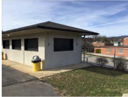
2). West Elevation - Feb 23, 2017
