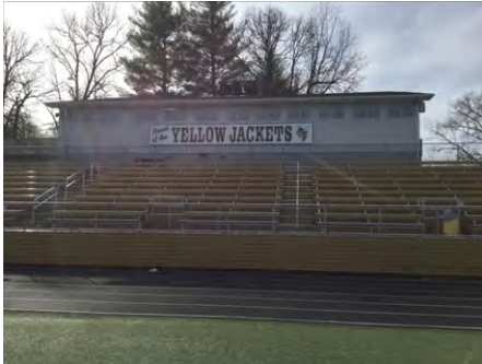
1). East Elevation - Feb 27, 2017
