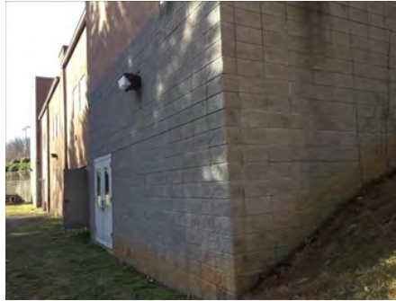
2). East Elevation - Feb 08, 2017
