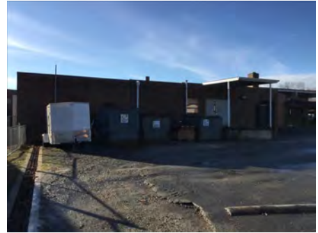
3). North Elevation - Jan 24, 2017
