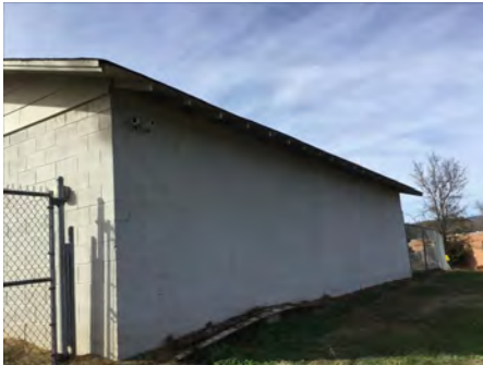
4). South Elevation - Feb 23, 2017
