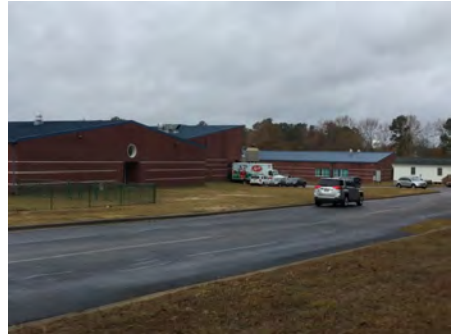
3). North Elevation - Dec 07, 2016
