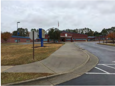
1). South Elevation - Dec 07, 2016
