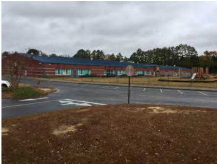
4). East Elevation - Dec 07, 2016
