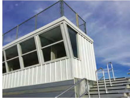
2). Southwest Elevation - Jan 24, 2017
