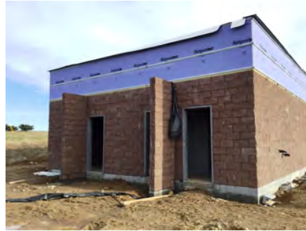
2). North Elevation - Jan 24, 2017
