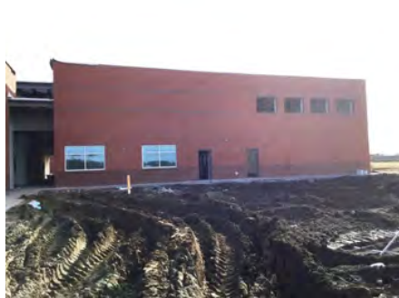
2). North Elevation - Jan 24, 2017
