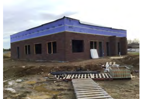
3). Northwest Elevation - Jan 24, 2017
