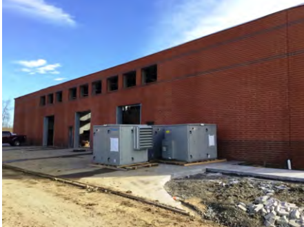
1). Northwest Elevation - Jan 24, 2017
