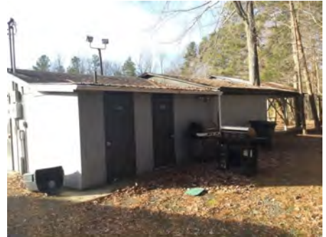
3). North Elevation - Feb 10, 2017
