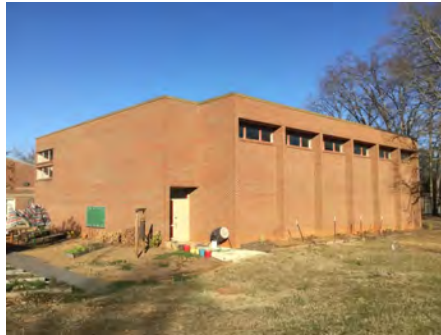
5). Southwest Elevation, Gym - Feb 10, 2017
