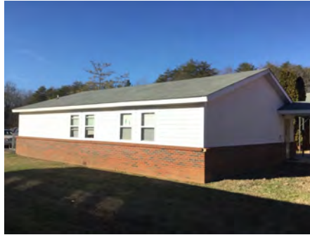
2). Southeast Elevation - Feb 10, 2017
