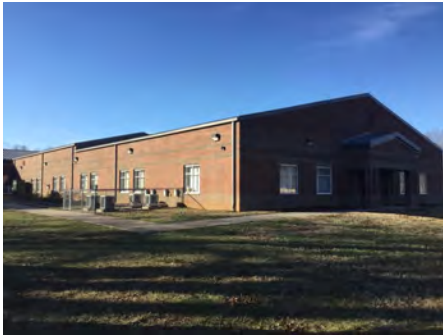
4). East Elevation - Feb 10, 2017
