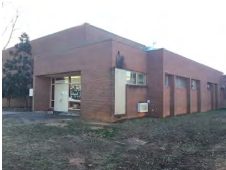
7). Northeast Elevation, Gym - Feb 10, 2017
