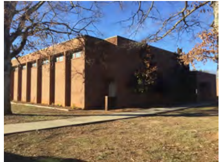
6). Southeast Elevation, Gym - Feb 10, 2017
