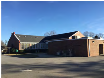
2). North Elevation, 1940 Bldg - Feb 10, 2017
