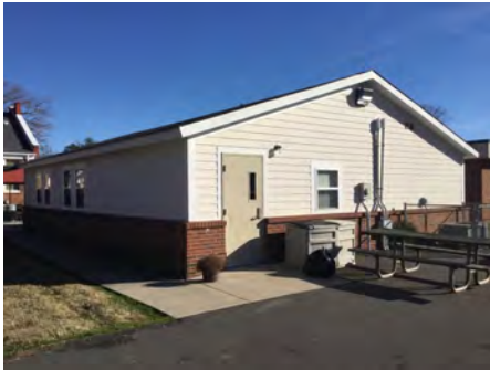
4). Northwest Elevation - Feb 10, 2017
