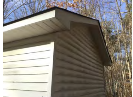
3). North Elevation - Feb 10, 2017
