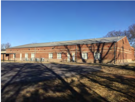
1). West Elevation - Feb 10, 2017
