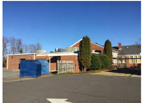
3). West Elevation, 1940 Bldg - Feb 10, 2017
