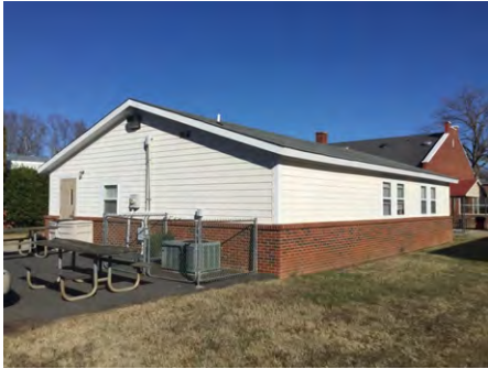
1). Southwest Elevation - Feb 10, 2017
