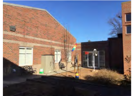
3). Southeast Elevation - Feb 10, 2017
