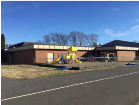
4). West Elevation, Media - Feb 10, 2017
