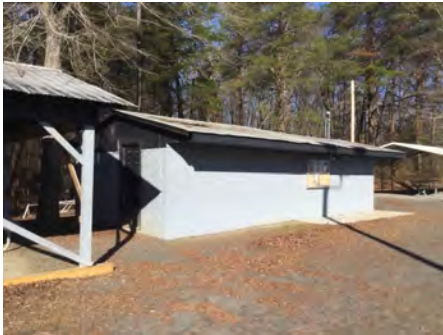
4). Southwest Elevation - Feb 10, 2017
