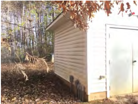
4). West Elevation - Feb 10, 2017
