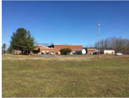
2). South Elevation - Feb 11, 2017
