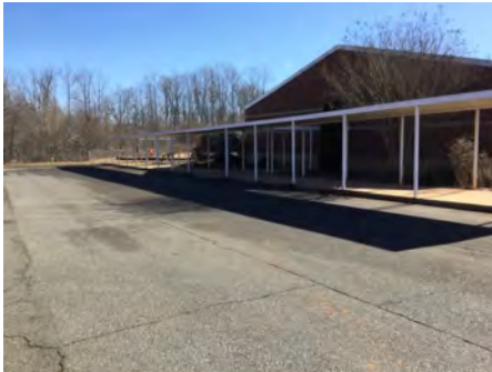
4). North Elevation - Feb 11, 2017
