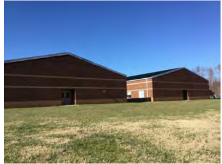
3). East Elevation - Feb 11, 2017
