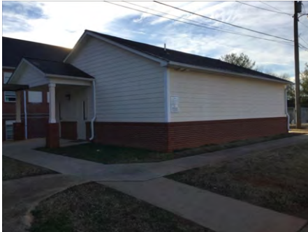
1). Northwest Elevation - Feb 10, 2017
