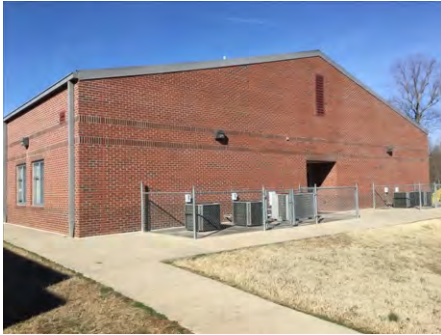
1). East Elevation - Feb 09, 2017
