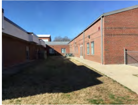
2). South Elevation - Feb 09, 2017
