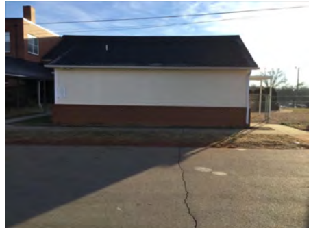
3). West Elevation - Feb 10, 2017
