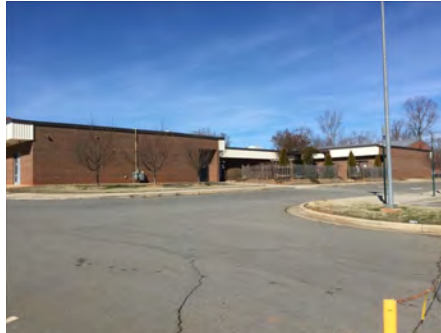
2). East Elevation - Feb 09, 2017
