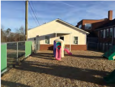
4). South Elevation - Feb 10, 2017
