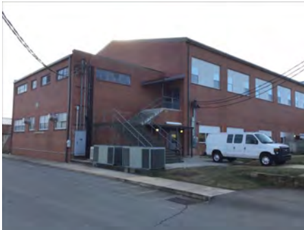
4). Northwest Elevation - Feb 09, 2017
