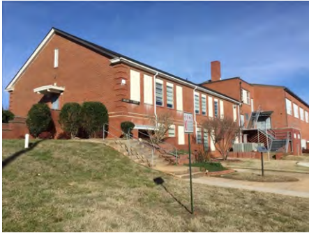
1). Southeast Elevation - Feb 09, 2017
