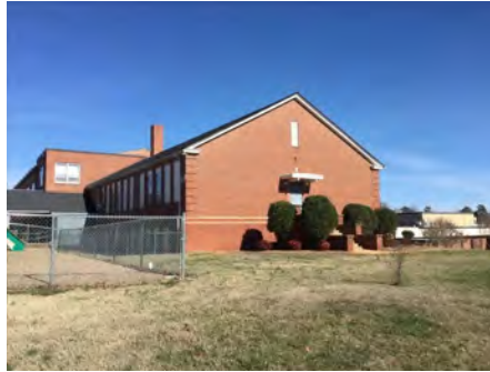
2). Southwest Elevation - Feb 09, 2017
