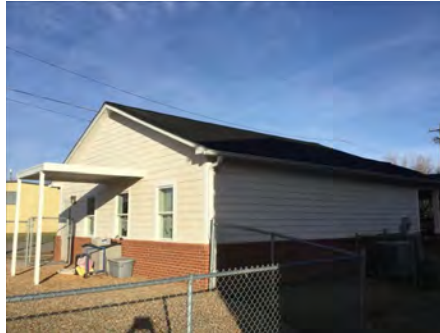
2). Southeast Elevation - Feb 10, 2017
