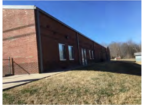
3). North Elevation - Feb 09, 2017
