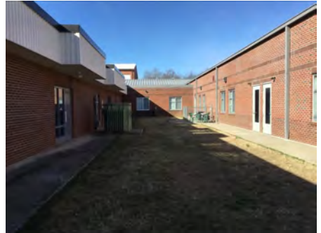
3). North Elevation - Feb 09, 2017
