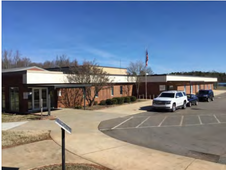
1). South Elevation - Feb 09, 2017
