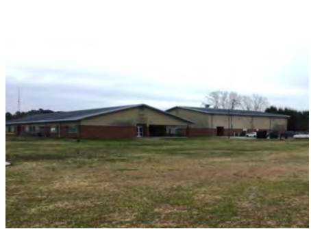
3). Northwest Elevation - Feb 06, 2017
