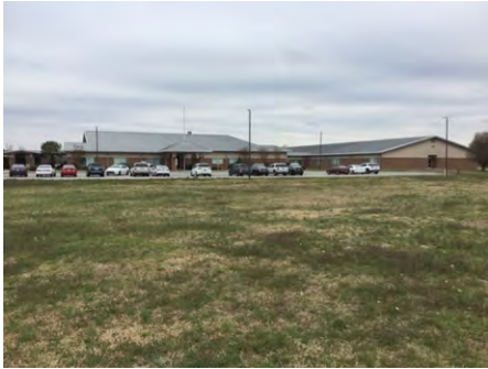
1). Southeast Elevation - Feb 06, 2017
