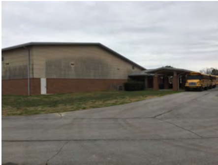
4). Southwest Elevation - Feb 06, 2017
