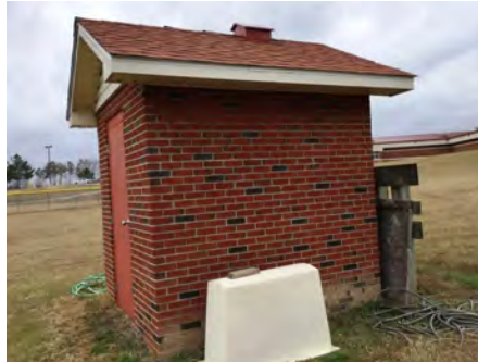
2). Northeast Elevation - Nov 29, 2016
