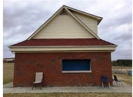
3). Northeast Elevation - Nov 29, 2016
