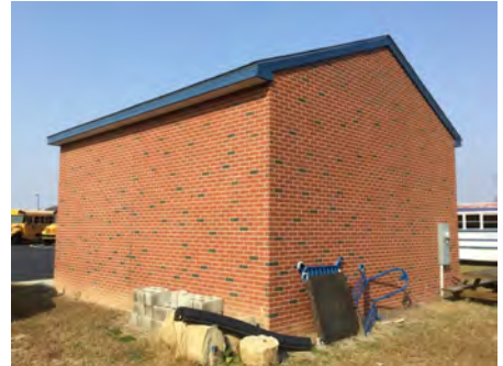
3). East Elevation - Dec 05, 2016
