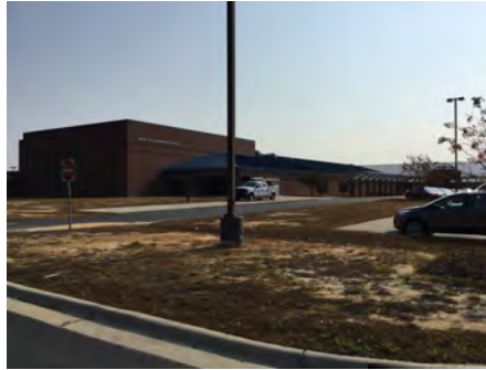
2). North Elevation - Dec 05, 2016
