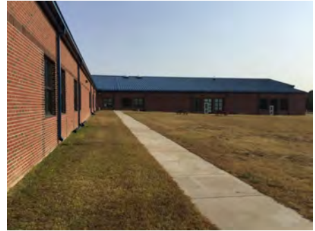
3). South Elevation - Dec 05, 2016
