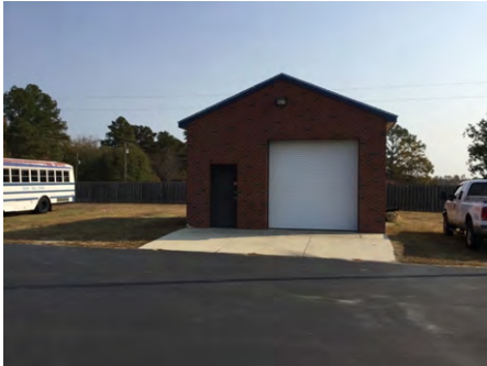
1). West Elevation - Dec 05, 2016
