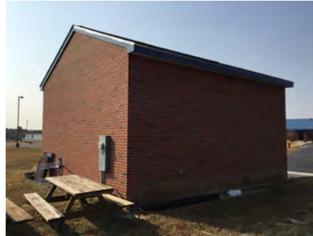
2). South Elevation - Dec 05, 2016
