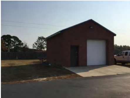
4). North Elevation - Dec 05, 2016
