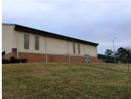
2). Southwest Elevation - Jan 19, 2017
