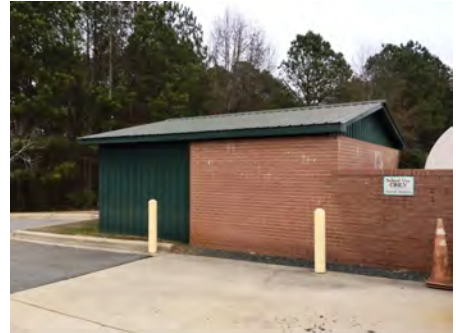
3). Southwest Elevation - Jan 19, 2017
