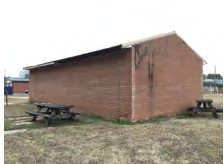
3). Southeast Elevation - Feb 06, 2017
