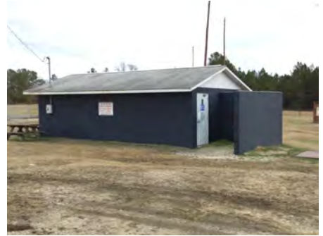
3). Southwest Elevation - Feb 06, 2017
