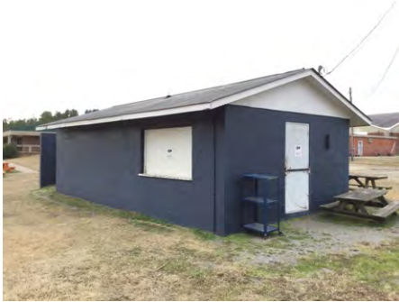
1). Northeast Elevation - Feb 06, 2017
