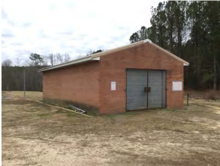
1). Northwest Elevation - Feb 06, 2017
