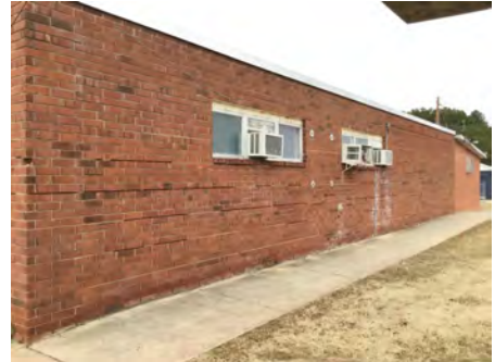
3). East Elevation - Feb 06, 2017
