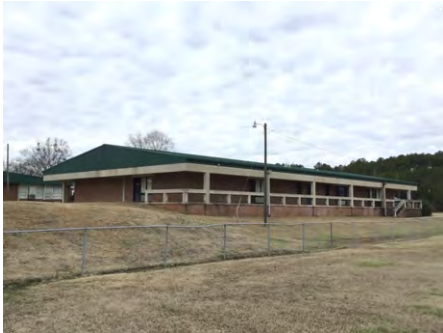
1). East Elevation - Feb 06, 2017
