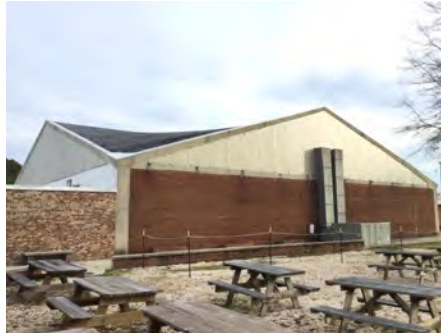
2). South Elevation - Feb 06, 2017
