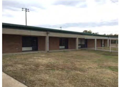
3). West Elevation - Feb 06, 2017
