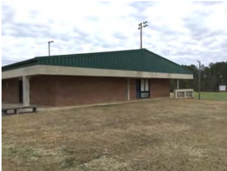
4). South Elevation - Feb 06, 2017
