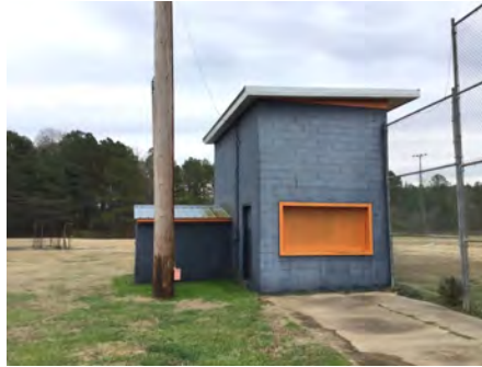
2). West Elevation - Feb 06, 2017
