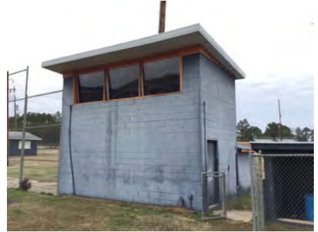
3). South Elevation - Feb 06, 2017
