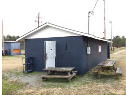
2). Northwest Elevation - Feb 06, 2017
