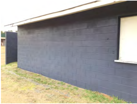
4). East Elevation - Feb 06, 2017
