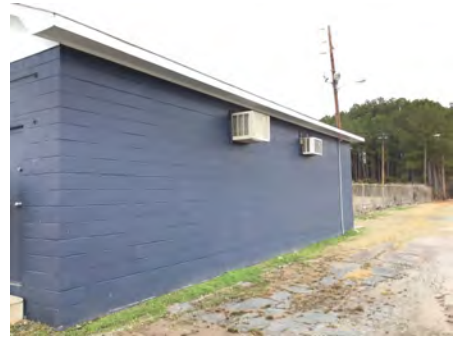
3). East Elevation - Feb 06, 2017
