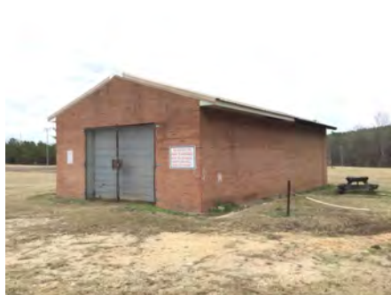
2). Southwest Elevation - Feb 06, 2017
