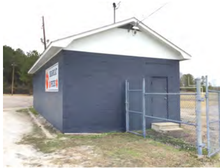
2). South Elevation - Feb 06, 2017
