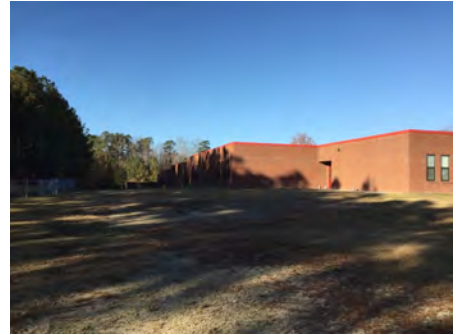
3). South Elevation - Dec 08, 2016
