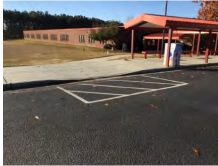
2). East Elevation - Dec 08, 2016
