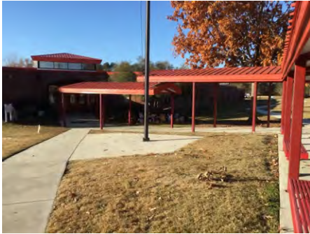
1). North Elevation - Dec 08, 2016
