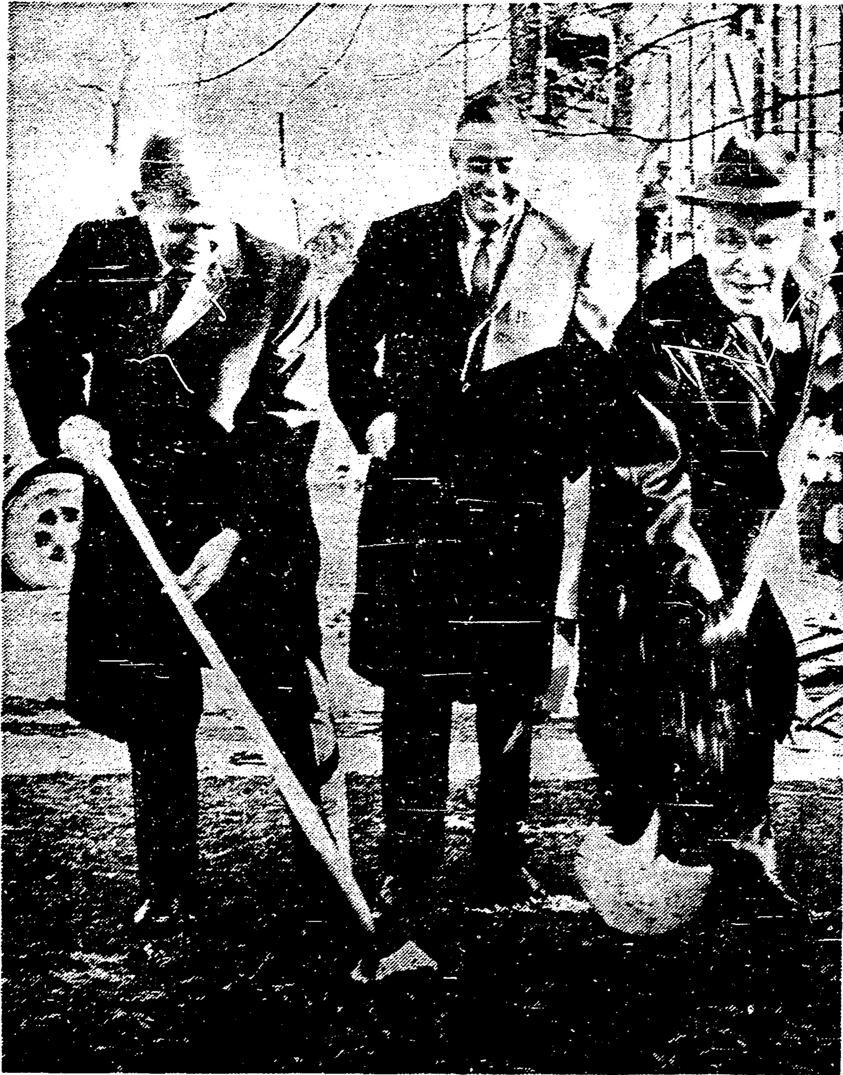
GROUND-BREAKERS TERRY SANFORD (L) AND LUTHER HODGES ... With Tom White, chairman of the Legislative Building Commission.
